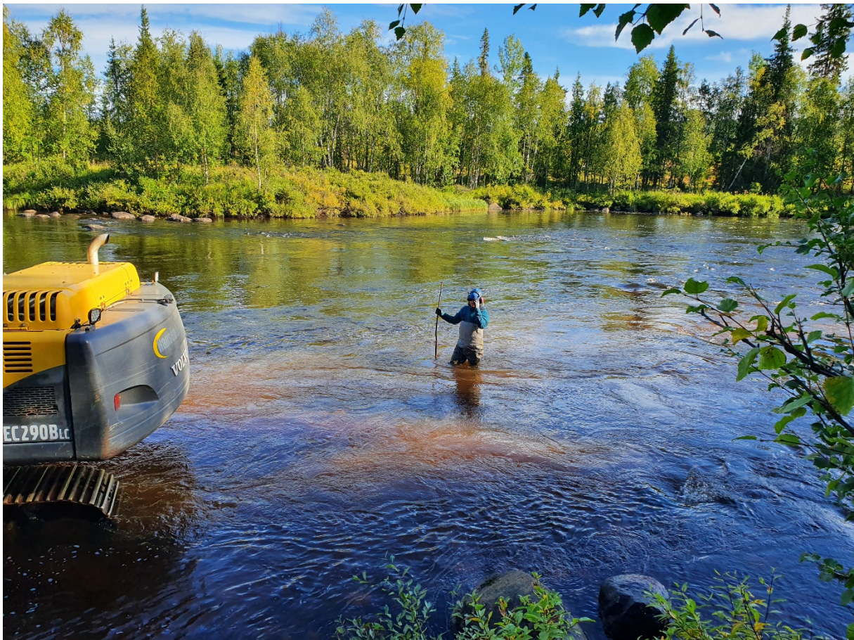
Picture 5. Adjusting spawning site one year after construction with mobile excavator unit and crew in Linaälven (project area Kalixälven). Area was used by salmon in autumn of 2021.
