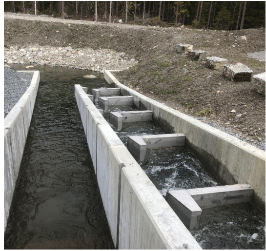
A constructed fish ladder in the upper part of River Bilstaån. Photo: Patrik Olofsson, CABN
