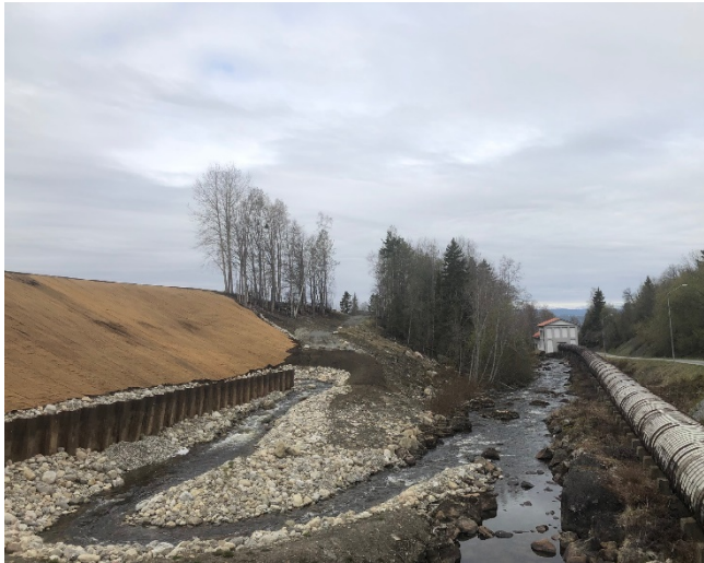
A constructed bypass channel in Bilstaån to secure fish migration past the first hydropower plant. Photo: Patrik Olofsson, CABN
