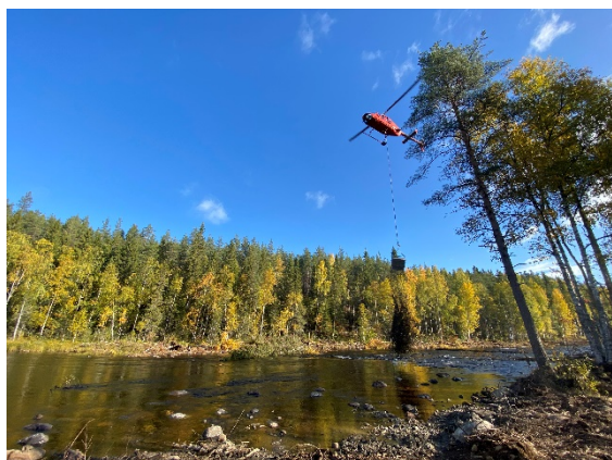
Picture 1. Helicopter, gravel to Lögdån 2020
