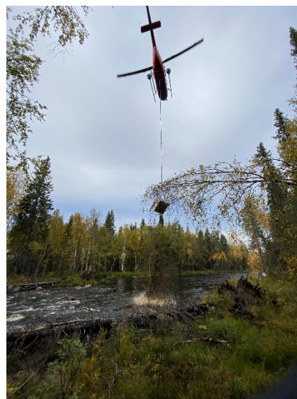
Picture 2. Helicopter, gravel to Lögdån 2020
