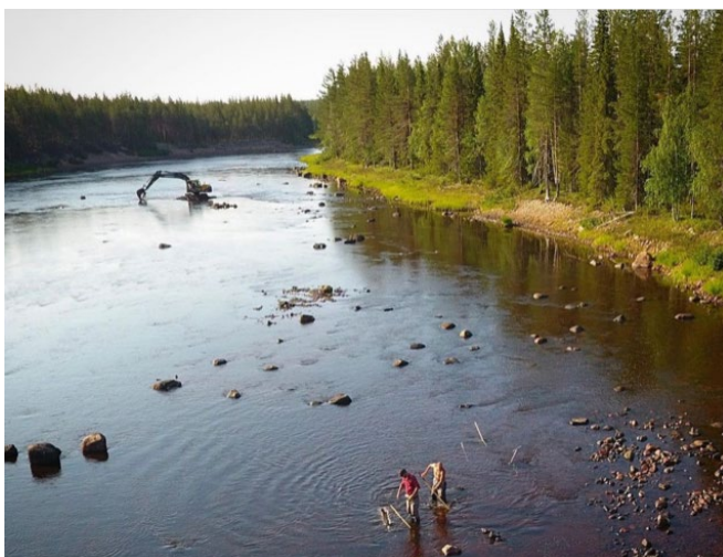
The service team is doing the final adjustment on a spawning bed and meanwhile the excavator is doing the preparation work for new spawning beds (project area Råneälven).
