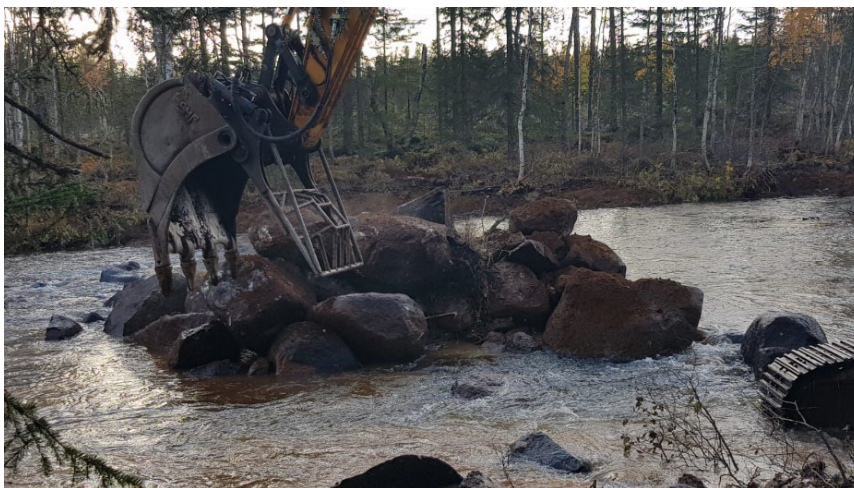
Excavator moving big boulders in project area Åbyälven.
